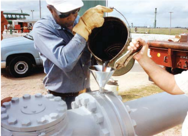
Flange filling is the process of pouring hot Innercoat between the flange faces to prevent corrosion.
