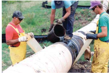
Innercoat wax coating being applied directly to the pipe surface using the Guard-Wrap wrapper as a "granny rag."
