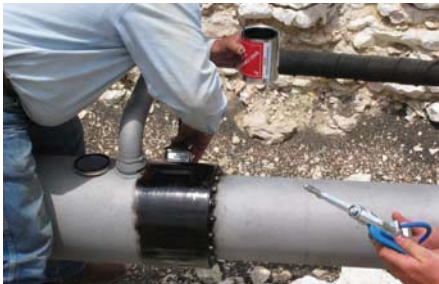
Seal-Wrap Primer being applied to the cleaned area of the casing.
