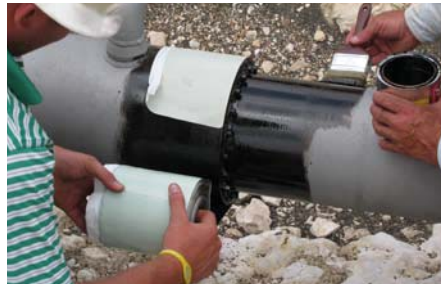
First layer of Double-Faced Adhesive is applied to the casing, Seal-Wrap Primer being applied to the carrier.
