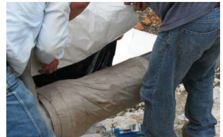
A second continuous wrap of Seal-Wrap applied directly over the first wrap.
