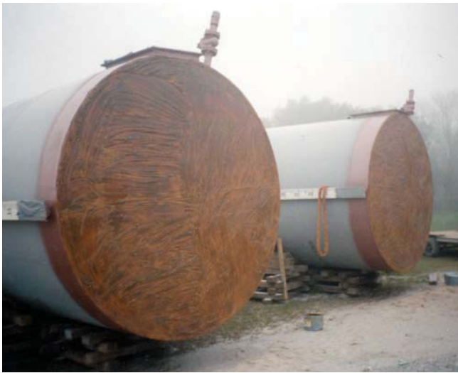
Temcoat applied to pipe surface. It will then be wrapped with Poly-Ply™, Guard-Wrap™ or Wax-Tape®.
