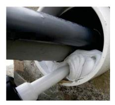
VISCOSEALANT: waterproofing cable and pipe penetrations. Left picture: sealing penetrations at vault system for control valves. Middle picture: multiple cables in one sleeve. Right picture: viscous elastic behavior during filling: the viscous component is dominant during filling and allows for flow around and in between the pipes, while the elastic component takes over when the material is in place; therefore no dripping or running can occur.
